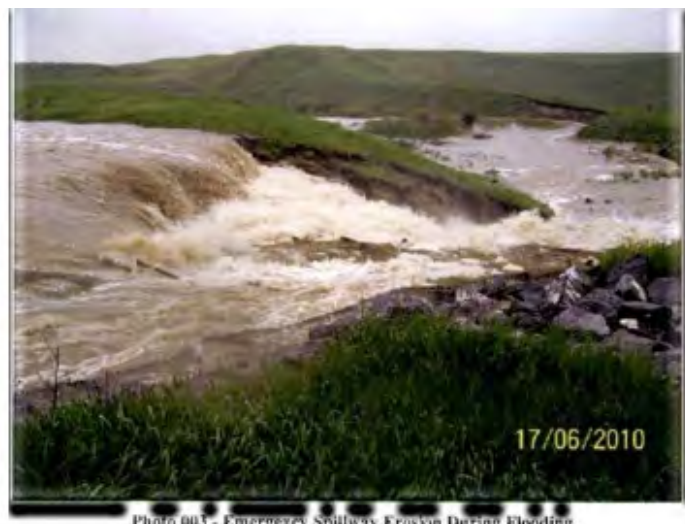
Photo 003 - Emergency Spillway Erosion During Flooding
