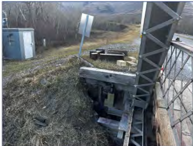
Nov. 13, 2025 Placing jack on the SW wing pile in preparation for pile stub repair
